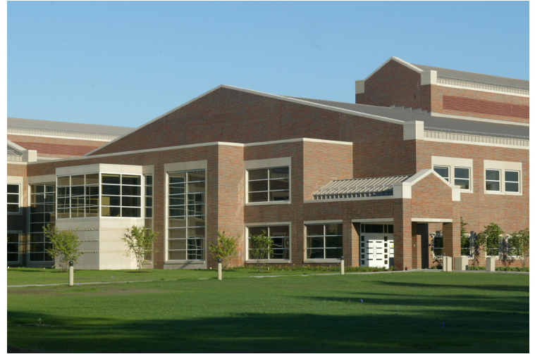
Central Michigan University's state-of-the-art Health Professions Building incorporates research, education, and clinical practice into one facility and facilitates sharing among faculty, students, researchers, and practitioners.
